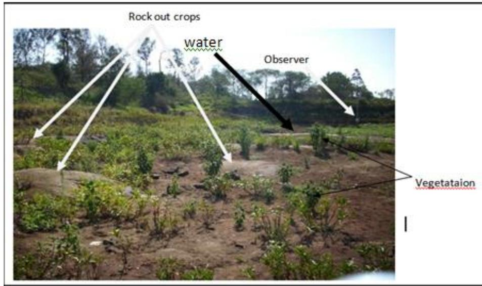
**Figure 5: The reservoir floor showing rock out crops that could be leakage outlets**
