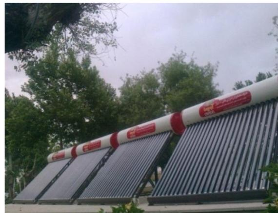
Figure 4. A solar collector mounted on the roof and adjusted to different tilt angles
